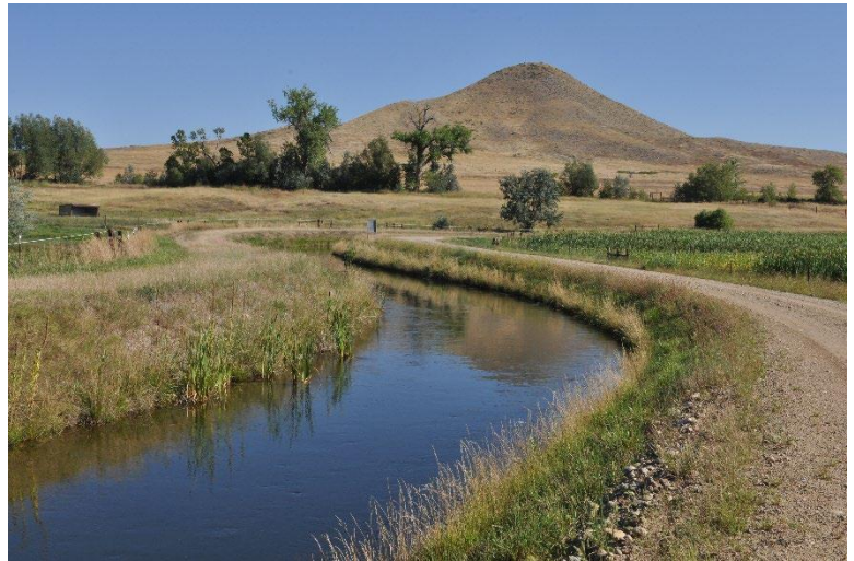
Boulder Feeder Canal.
