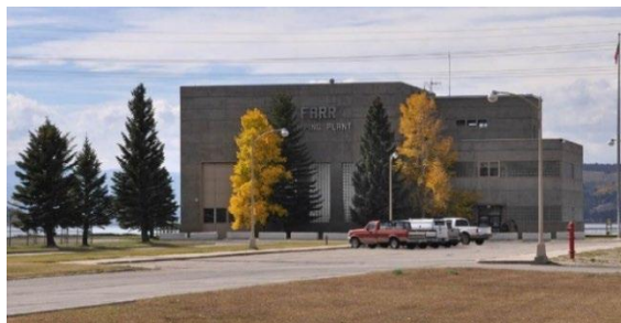
Farr Pump Plant
